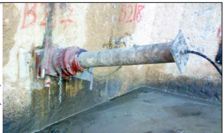
Installation of ground anchors
