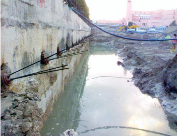
Groundwater within excavation (between dewatering stages)
