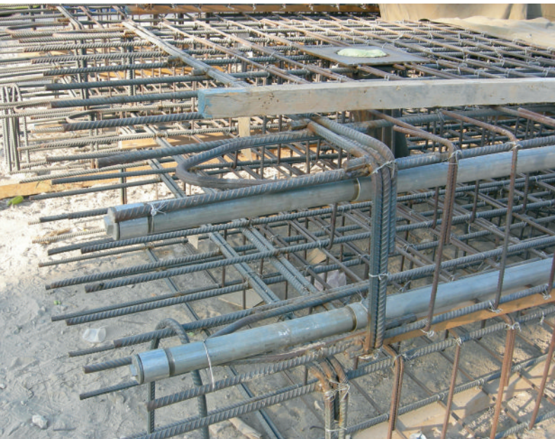
Steel reinforcement for diaphragm wall
