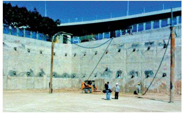
Conditions within excavation with pumps in operation
