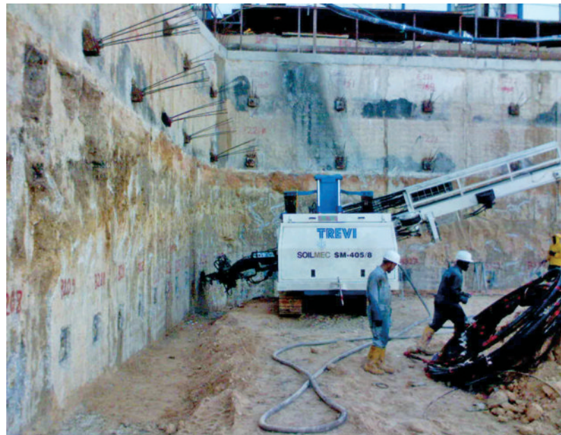
Installation of ground anchors
